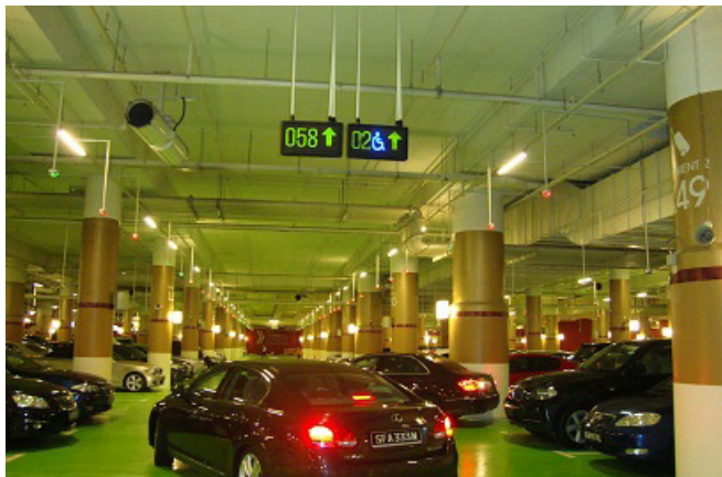
Fig. 37: Lowered sensor installation
