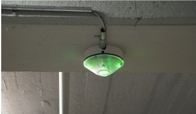
Fig. 36: Sensors mounted on the ceiling
