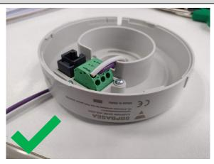
Leave some spare cable for each sensor (2/3 cm) in order to have enough cable to make the connection with the sensors connectors easier.
