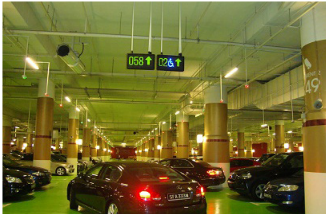
Fig. 36: Lowered sensor installation
