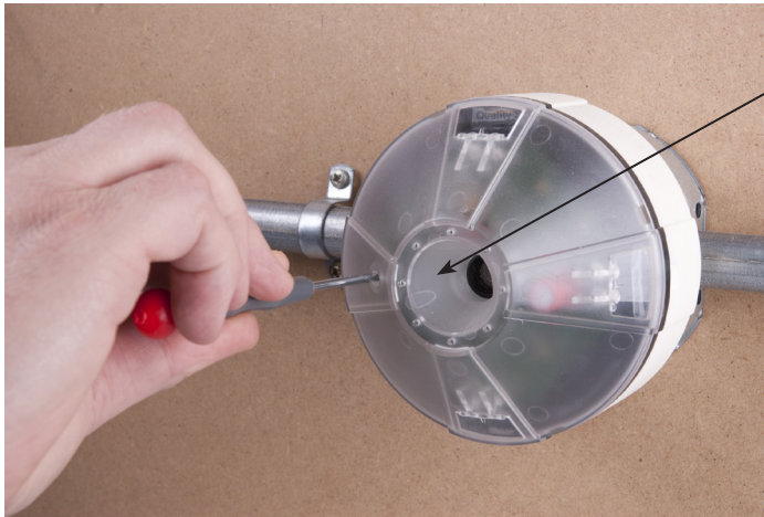
Fig. 27: Calibration of a sensor (local)
