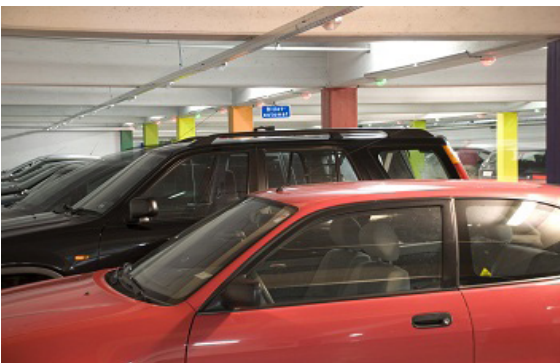
Fig. 34: Sensors mounted on a cable tray
