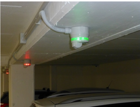
Lowered sensor installation
