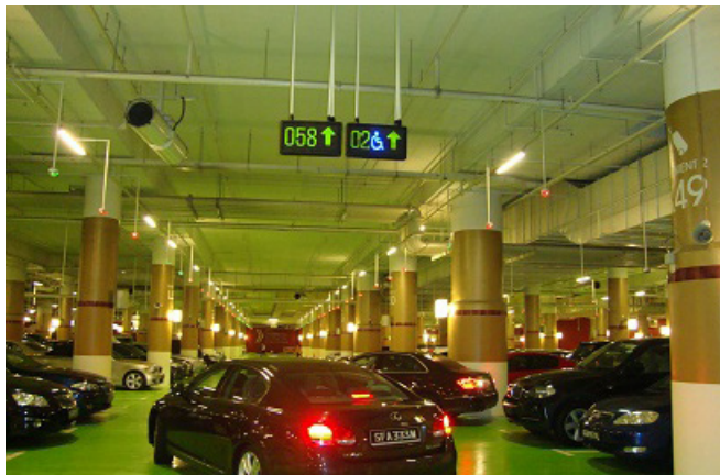
Fig. 36: Lowered sensor installation
