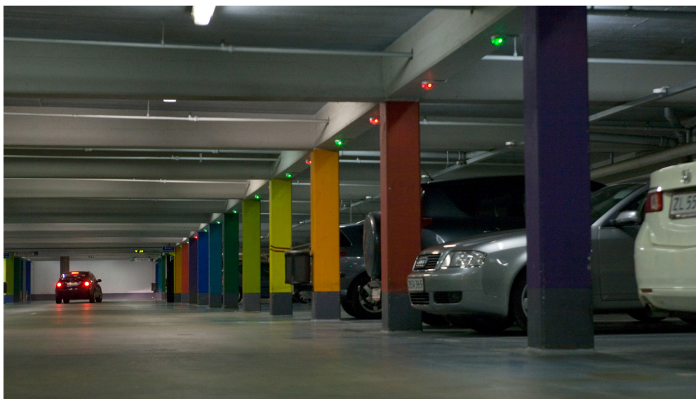
Fig. 18: Driveway with external indicator lights providing a clear view
